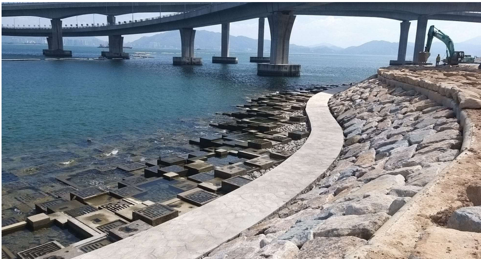
General View of Rocky Eco-shoreline
