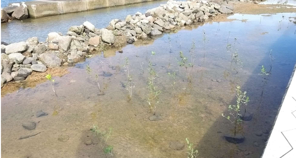
General View of Mangrove Eco-shoreline Upper Terrace
