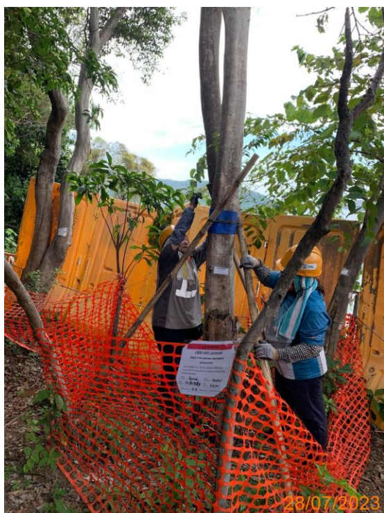
19: Installation of staking for U041
