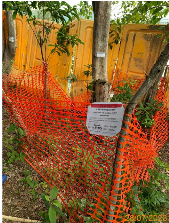
22: Temporary protective fencing for U041, U042 and U043
