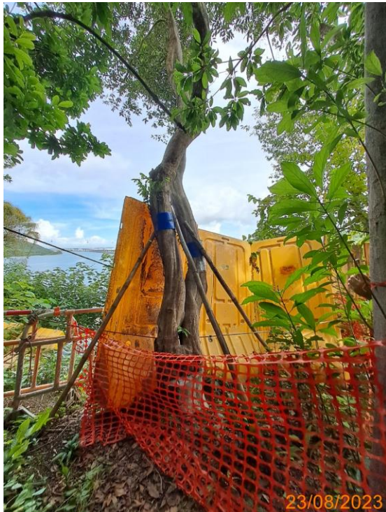
19: Temporary protective fencing for U041, U042 and U043
