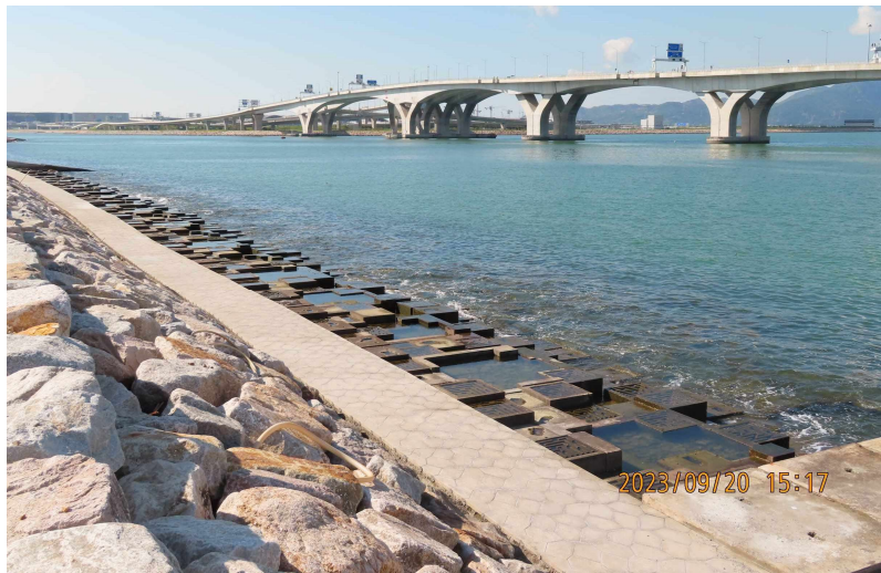
General View of Rocky Eco-shoreline
