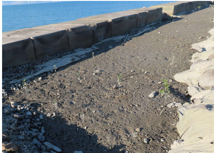
General View of Mangrove Eco-shoreline Lower Terrace
