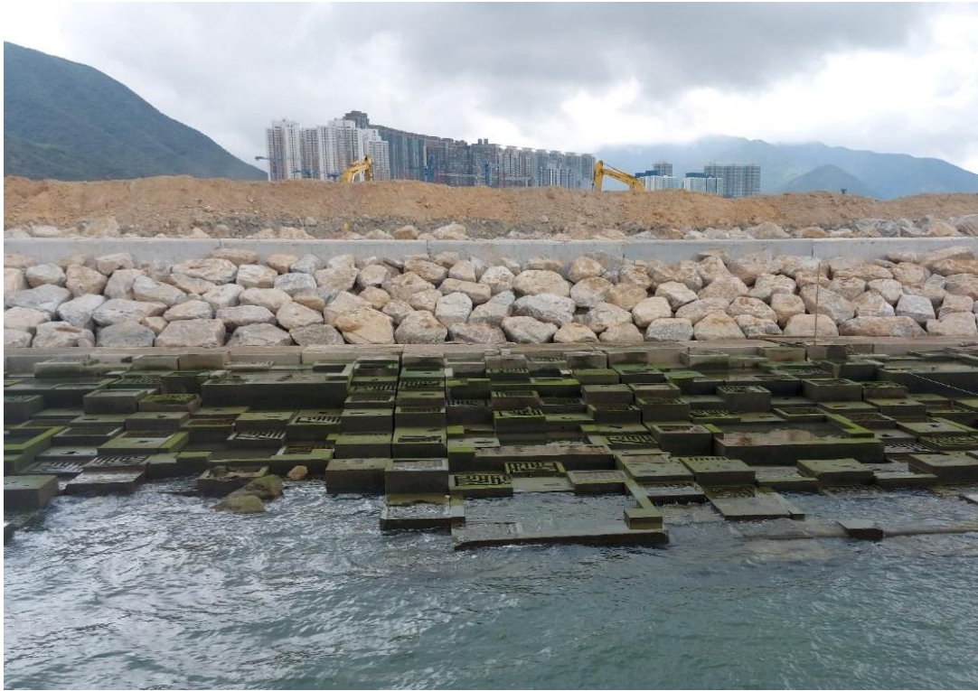
Photo 4 – Natural Rock Material/Planting for Artificial Seawall
