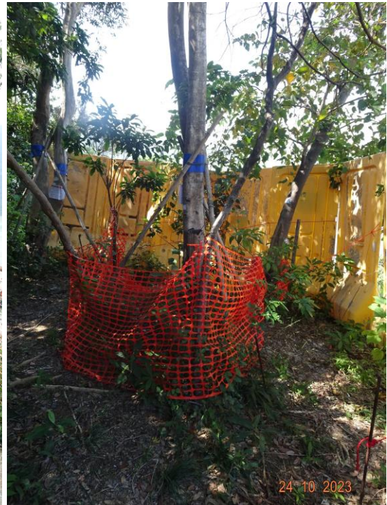
20: Temporary protective fencing for U041, U042 and U043
