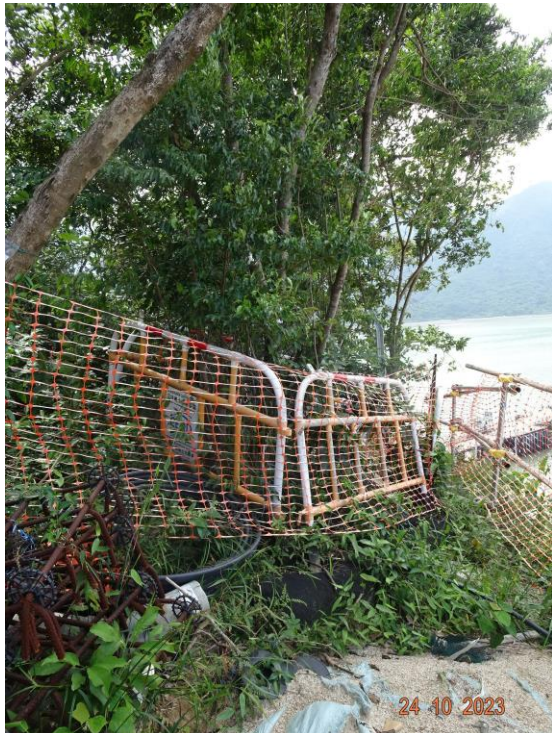
19: Silt rock and protection zone
