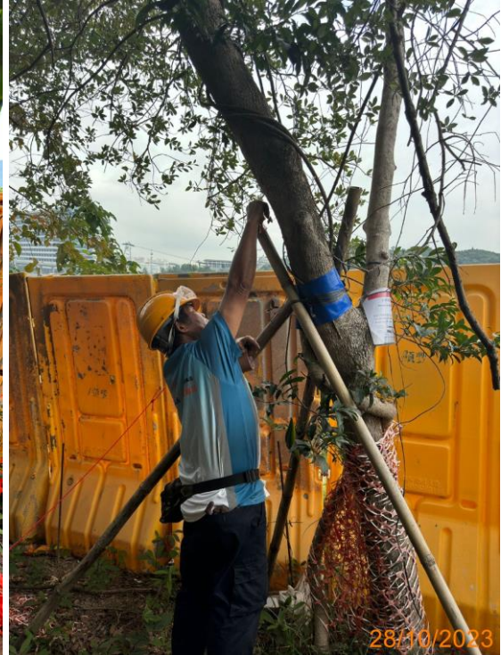
18: Readjustment of staking
