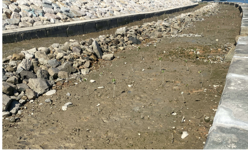
General View of Mangrove Eco-shoreline Lower Terrace
