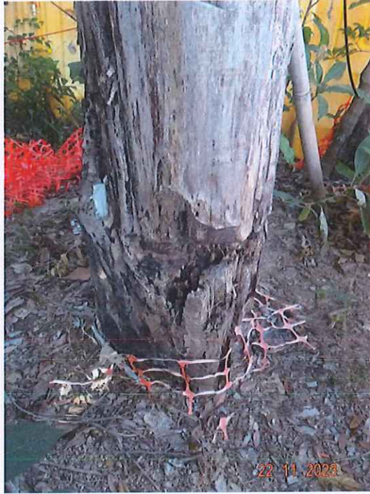
8: U041_Wood damaged by termite
