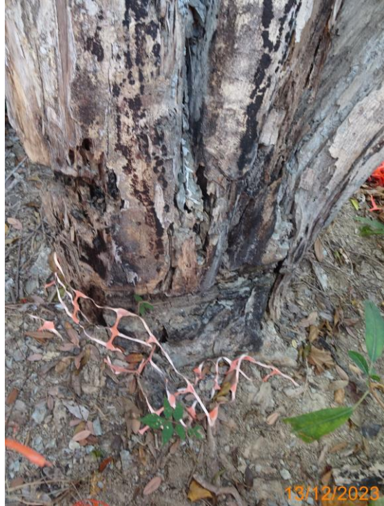
10: U041_ Wood damaged by termite
