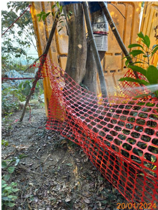
17: Spraying of termiticide
