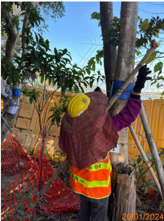
18: Re-adjustment of staking
