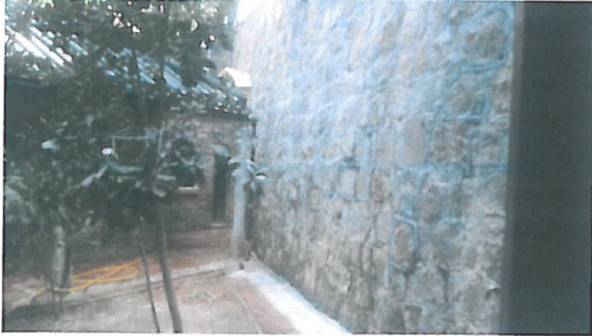
Photo 1 Taken on 23/12/2017 at Feature No.11SW-A/R94
