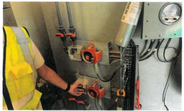
25ppm H2S Calibration for Inlet H2S Sensor
