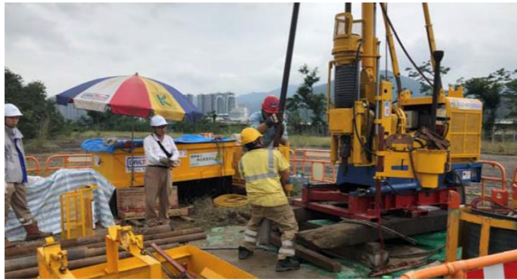
Borehole Drilling
