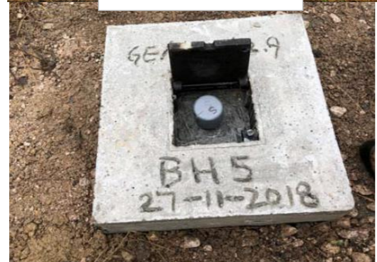
Installed GW Well
