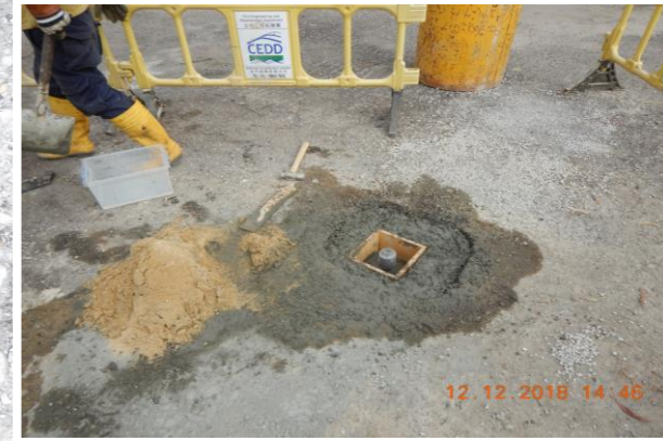
Set-up of Monitoring Well
