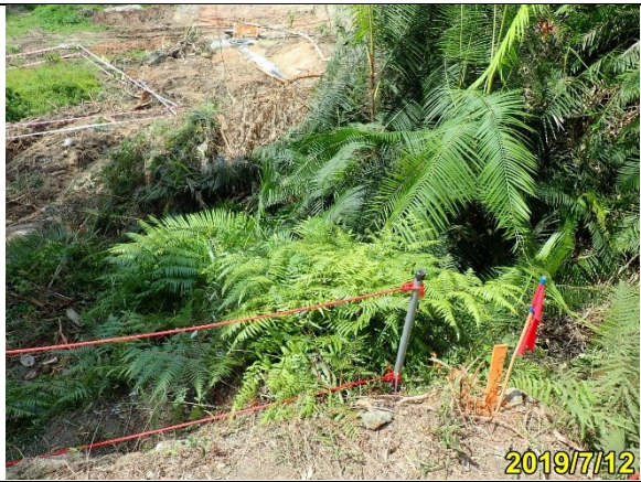
E0004 – Pre-construction survey
