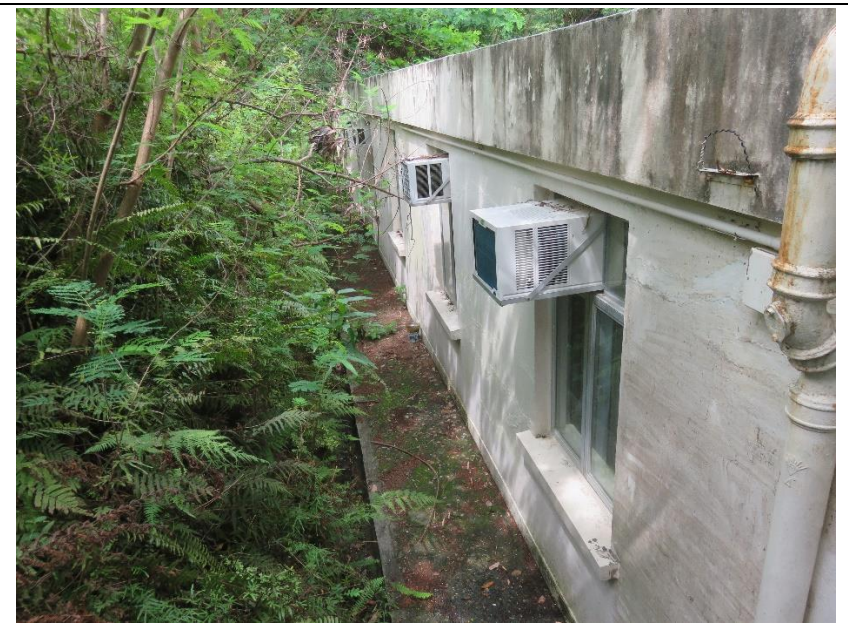
First Platform (Back of building)
