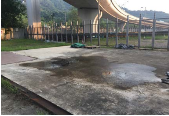
Photo 7: Spent Vehicle Batteries Storage Area at the south of Container Detention Area
