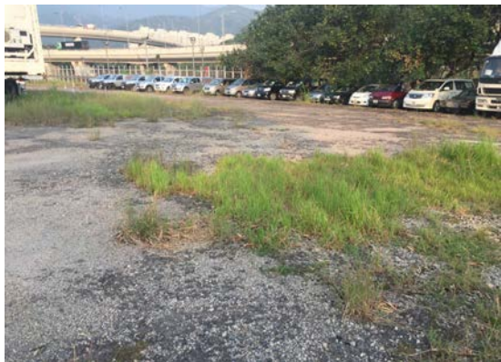
Photo 4: Motor Spirit Transfer Area at the southern end of Vehicle Detention
