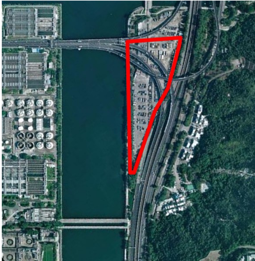
Year 2009(ref: CS25119, height: 6,000) – Overview of the C&ED Shatin VDC which the operation was commenced in 2004.
