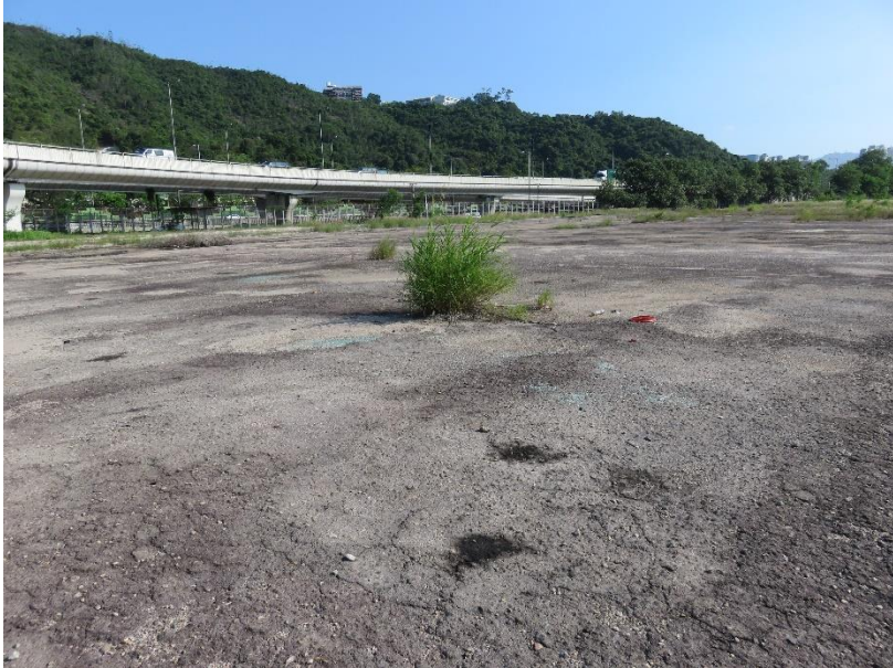
Engineer oil stain observed in recent walkover
