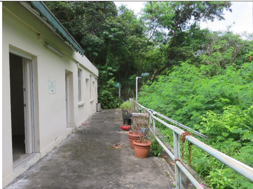
First Platform (Front of building)
