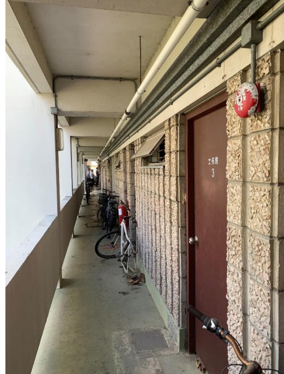
Photo 7 – Corridor of Block A, G/F
