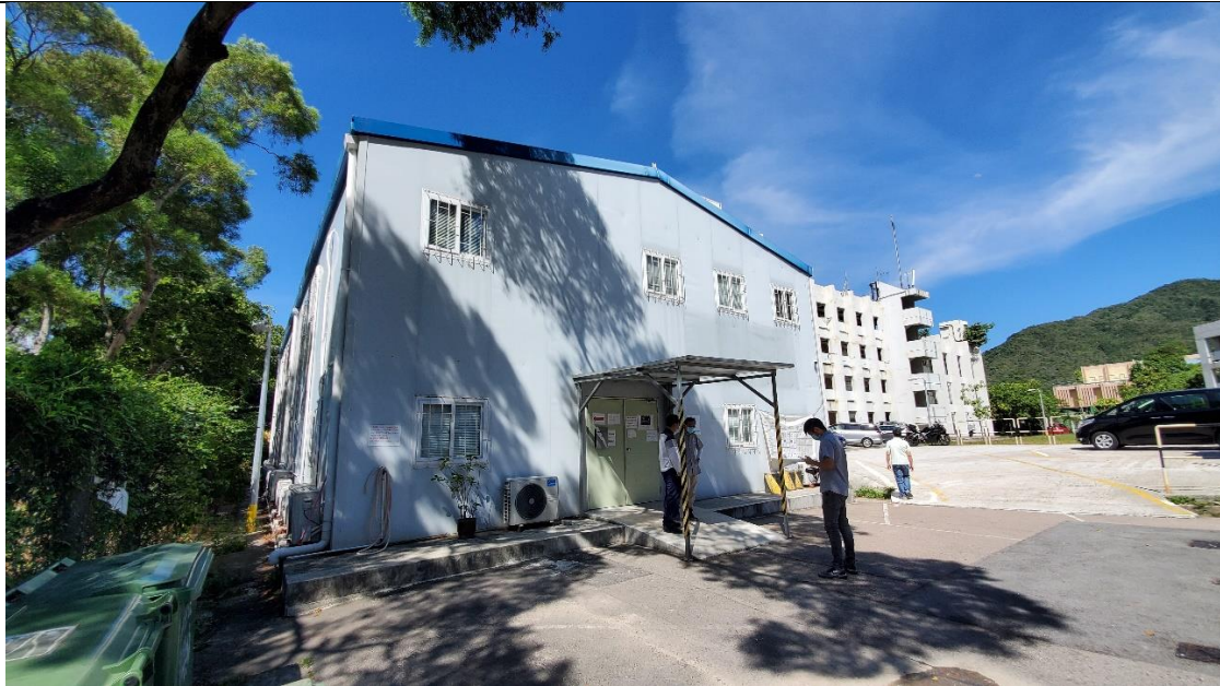
Photo 28 – Entrance of the Site Office
