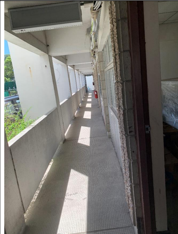
Photo 17 – Corridor, Block E, G/F
