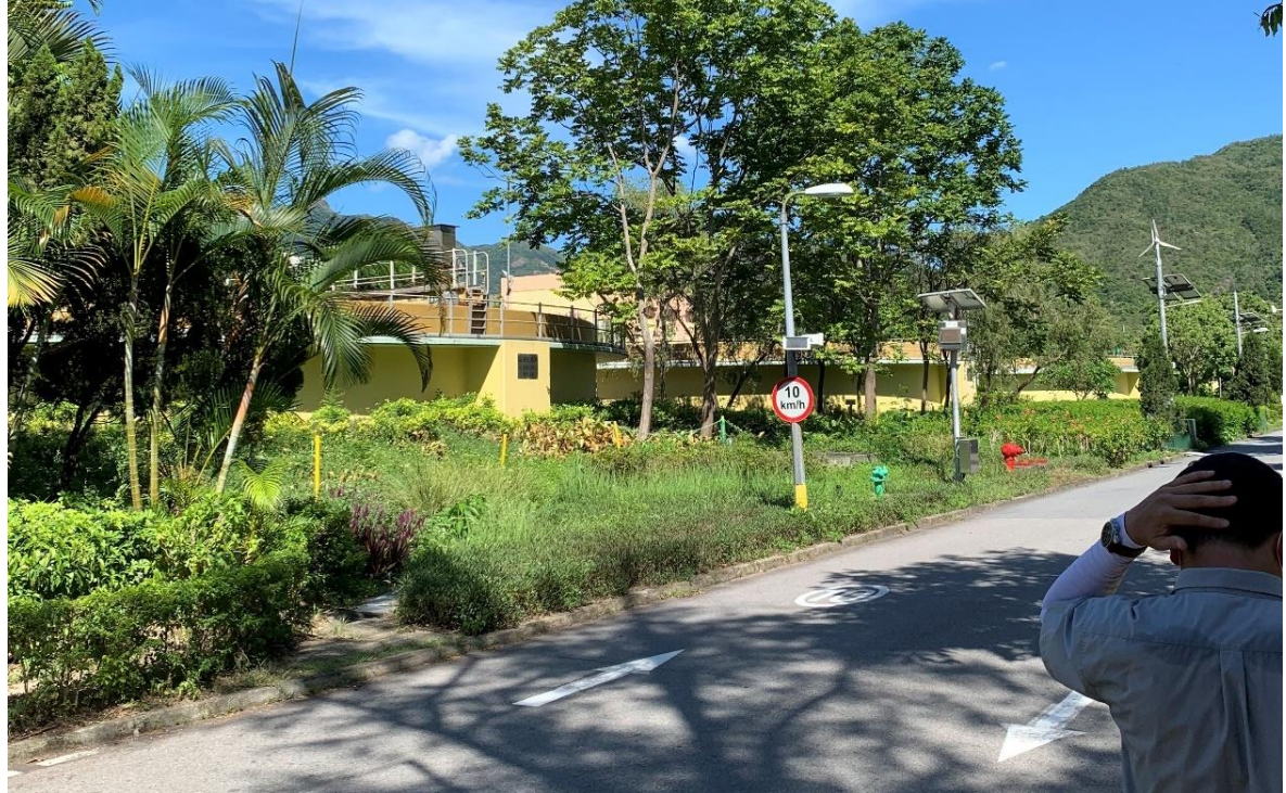
Photo 5 – Sha Tin Sewage Treatment Works at the northeast of the Site
