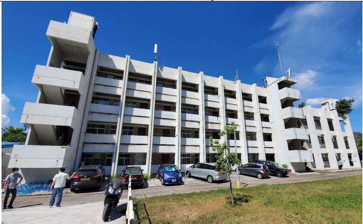
Photo 2 – DSD's Staff Quarter – Block D & E Southern Facade
