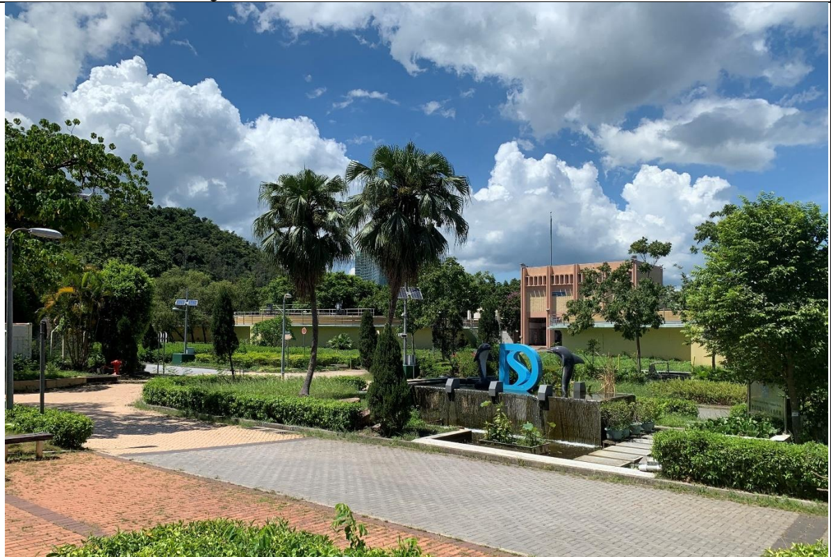
Photo 6 – Sha Tin Sewage Treatment Works at the east of the Site
