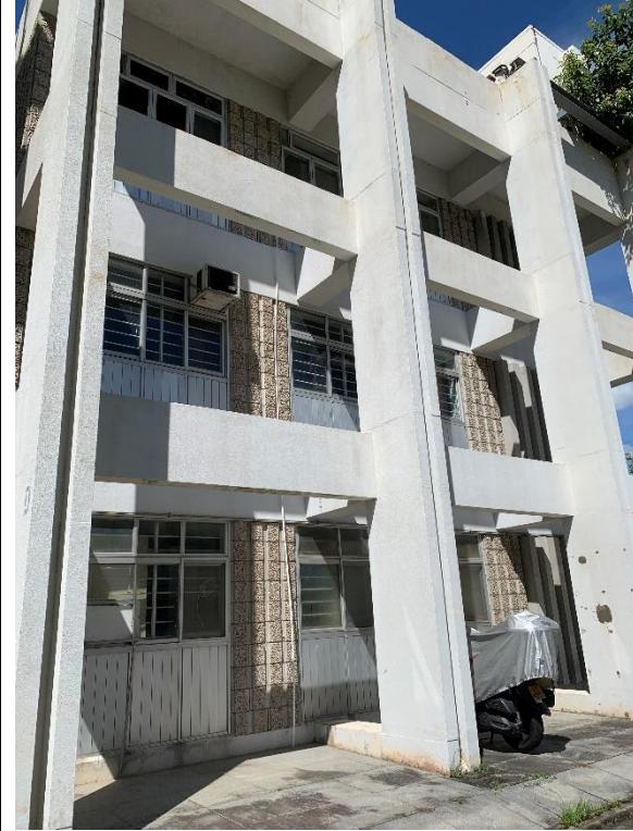
Photo 25 – Southern Façade of Block D, G/F
