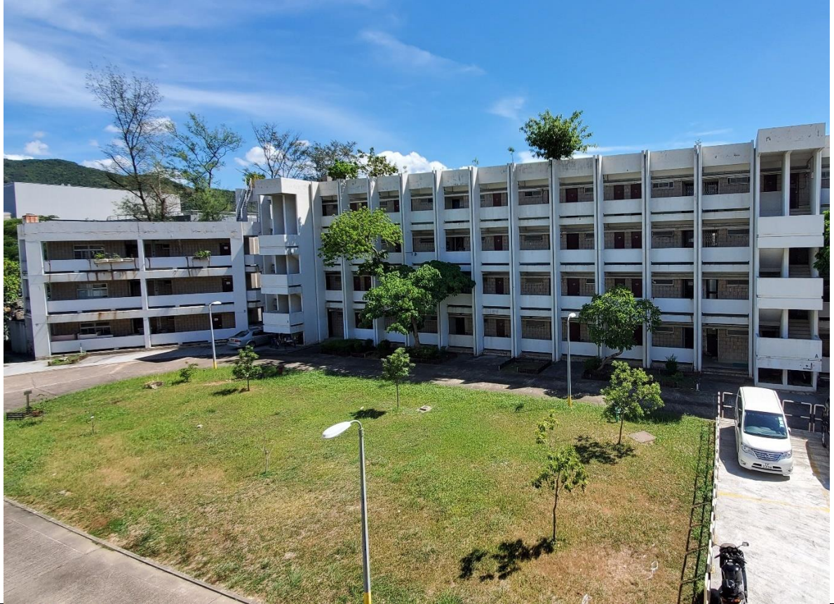
Photo 1 – DSD's Staff Quarter – Block A & B Northern Façade
