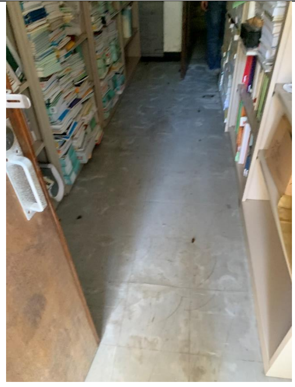
Photo 18 – Room 1, Block E, G/F
