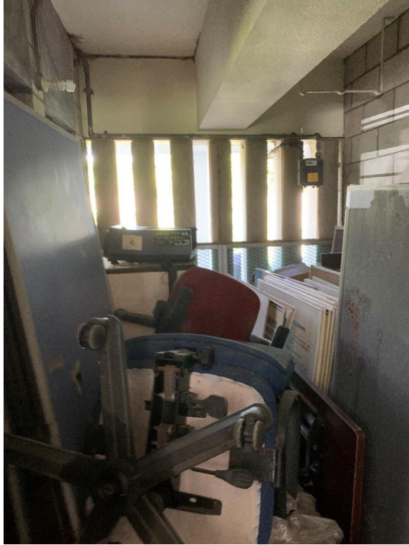
Photo 21 – Balcony of Room 4, Block E, G/F
