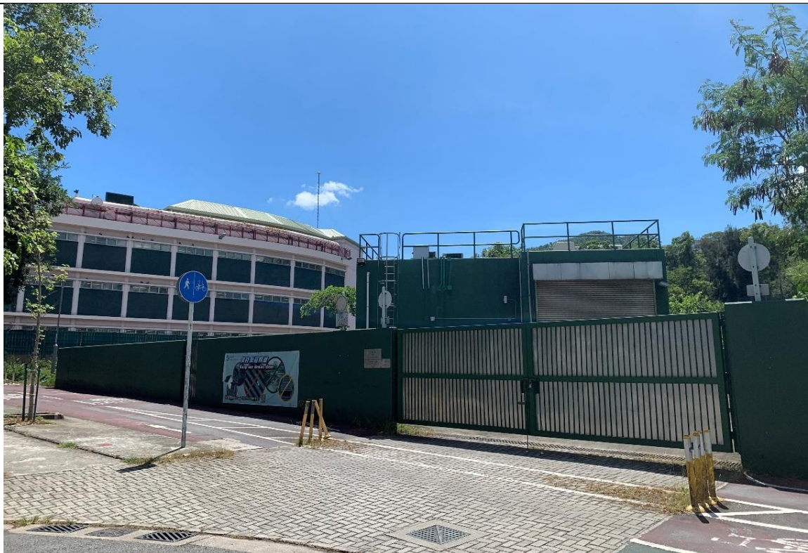
Photo 4 – DSD's Sewage Pumping Station at the northwest of the Site
