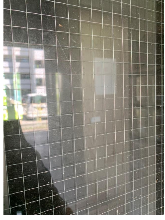
Photo 8 – Living Area at Block A, G/F
