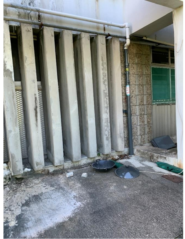
Photo 26 – Northern Façade of Balcony of Block D, G/F
