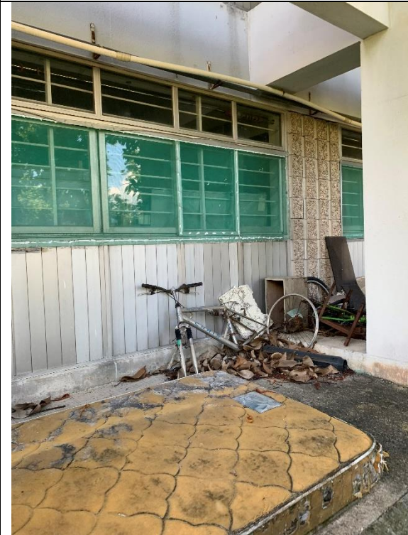
Photo 27 – Northern Façade of Living Area of Block D, G/F
