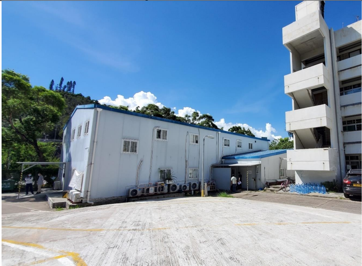
Photo 3 – Container Site Office for Contract DC/2017/02
