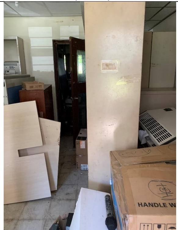
Photo 20 – Room 4, Block E, G/F
