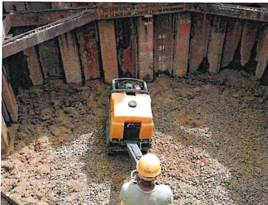
Backfilling of Zone 1 Treated Soil (Approx. From 1.13m bgl to 2.70m bgl)
