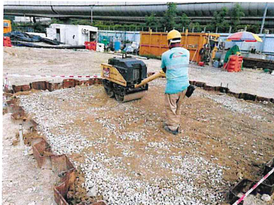
Backfilling of Clean Soil to Ground Level
