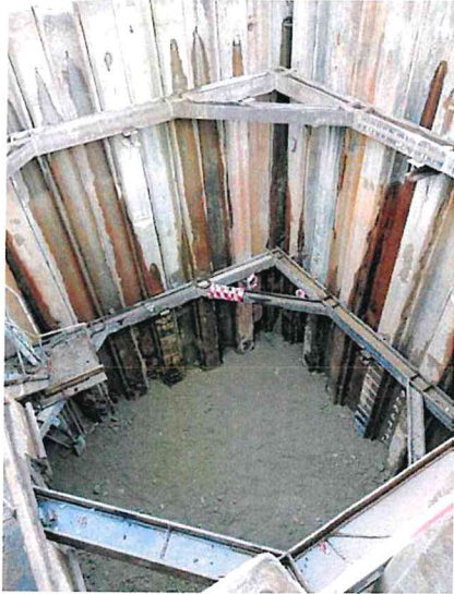
Backfilling of Zone 3 Treated Soil (Approx. From 4.73m bgl to 6.75m bgl)
