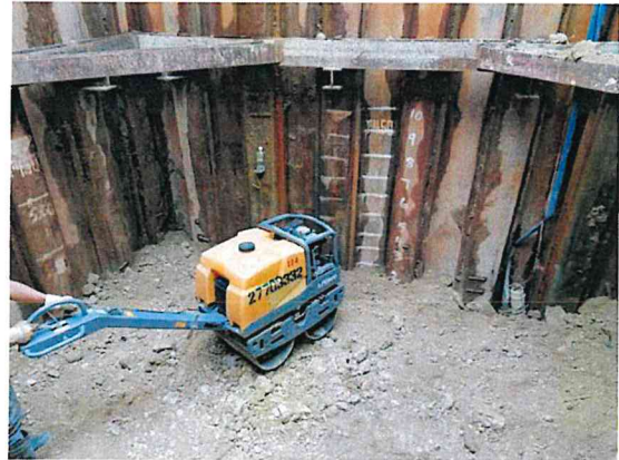
Backfilling of Zone 3 Treated Soil (Approx. From 4.73m bgl to 6.75m bgl)
