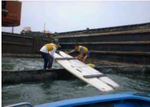
(a) maneuvering the wind-surfer boards over the silt curtain
