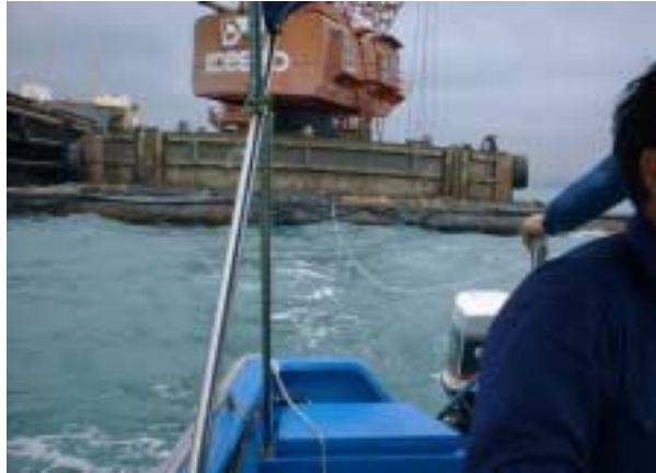
Figure 2.2 Hooking the rope to the edge of silt curtain
