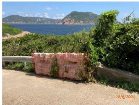
Collapsed fencing to be rectified
