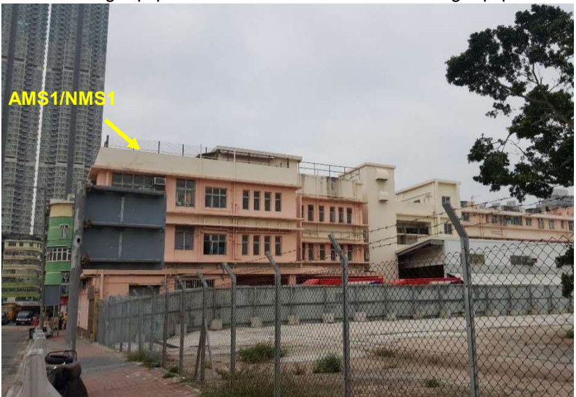
Overview of monitoring station AMS1/NMS1
