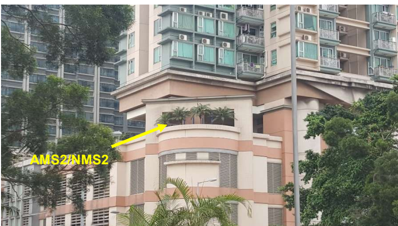
Overview of monitoring station AMS2/NMS2
