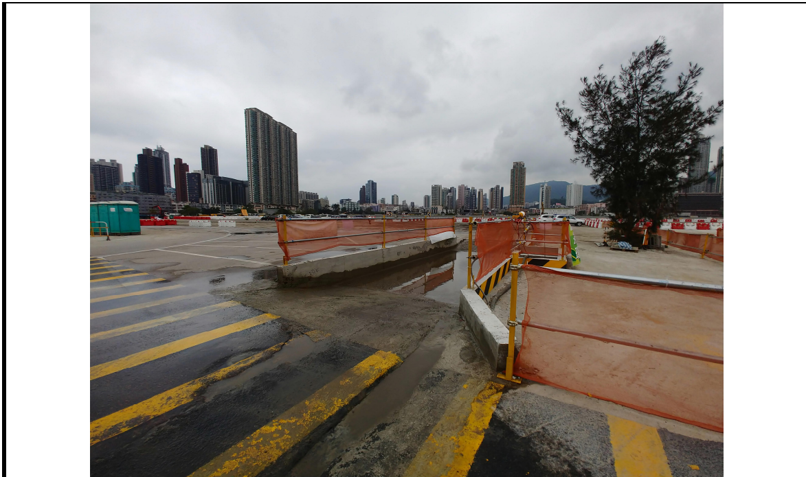
3. Wheel washing pool has been setup to minimize dust carried by leaving vehicles.
