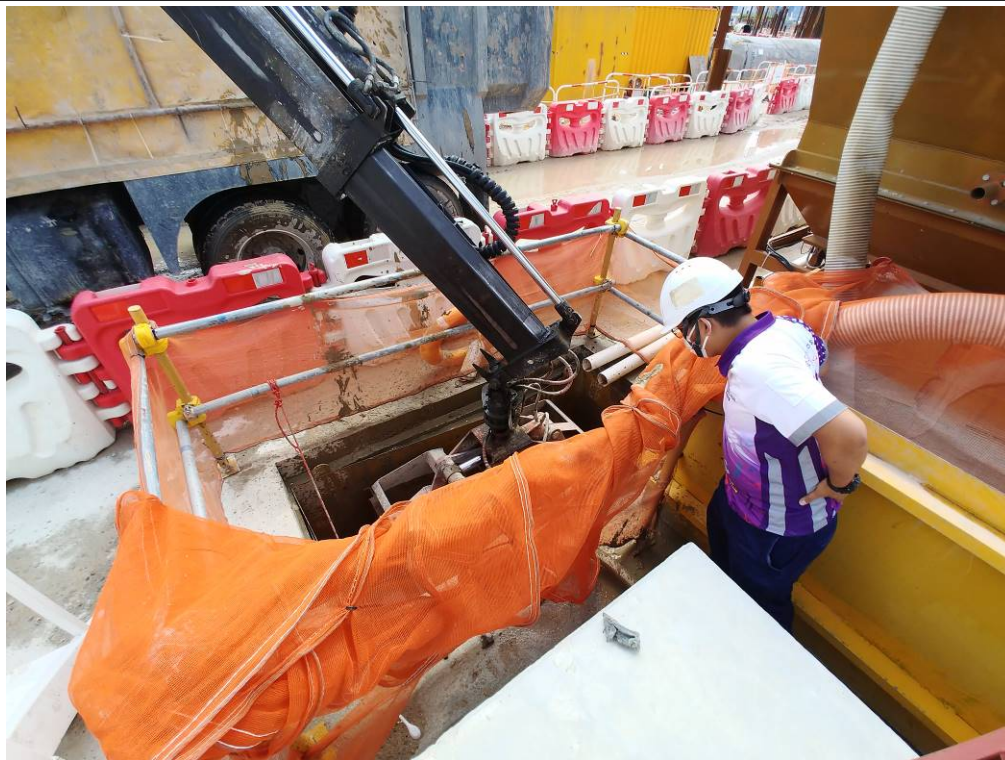
Photo 7b: Regular Sludge Removal at Wastewater Treatment Tank
