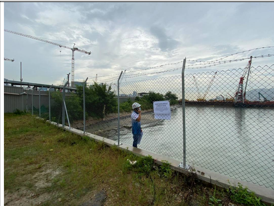
Photo 6b: Regular Checking at Sea Shore near Box Culvert
