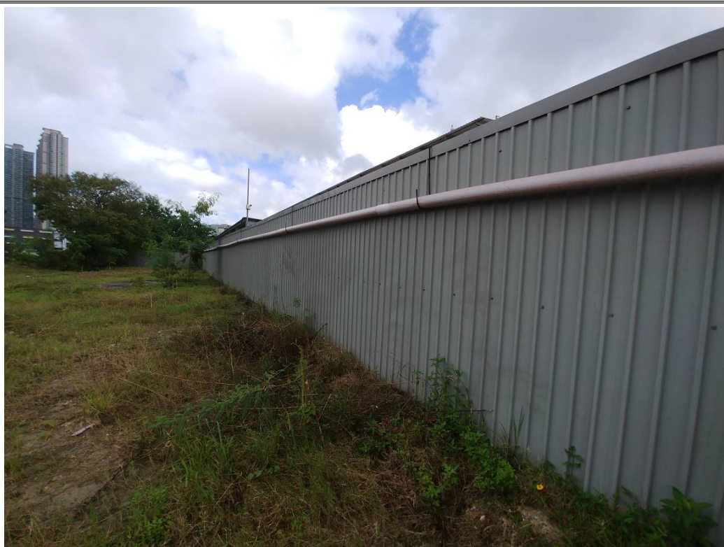
Photo 3: Site Hoarding near Seashore (16 September 2020)
