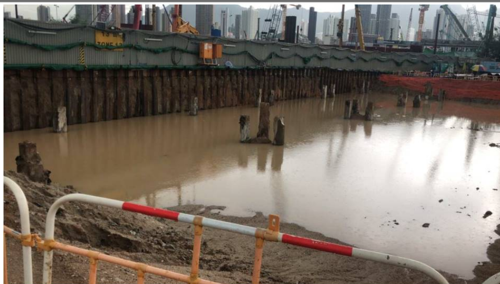
Photo 8a: Temporary Sedimentation Pond on Site
