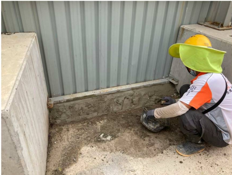
Photo 5: Re-sealing of Footing at Site Hoarding
