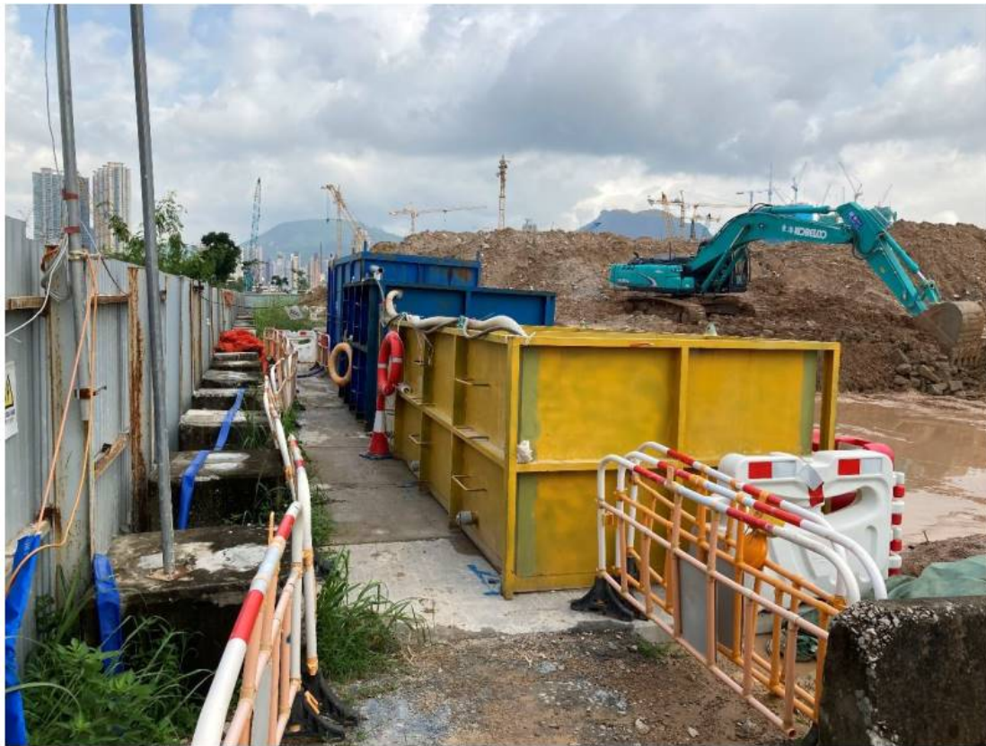
Photo 6: Provision of Sedimentation Tank for Temporary Storage of Wastewater on Site
