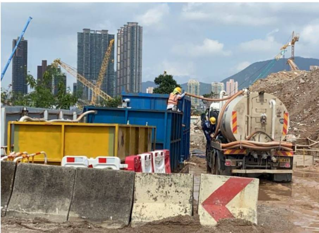
Photo 7: Regular Sludge Removal for the Sedimentation Tank on Site.
