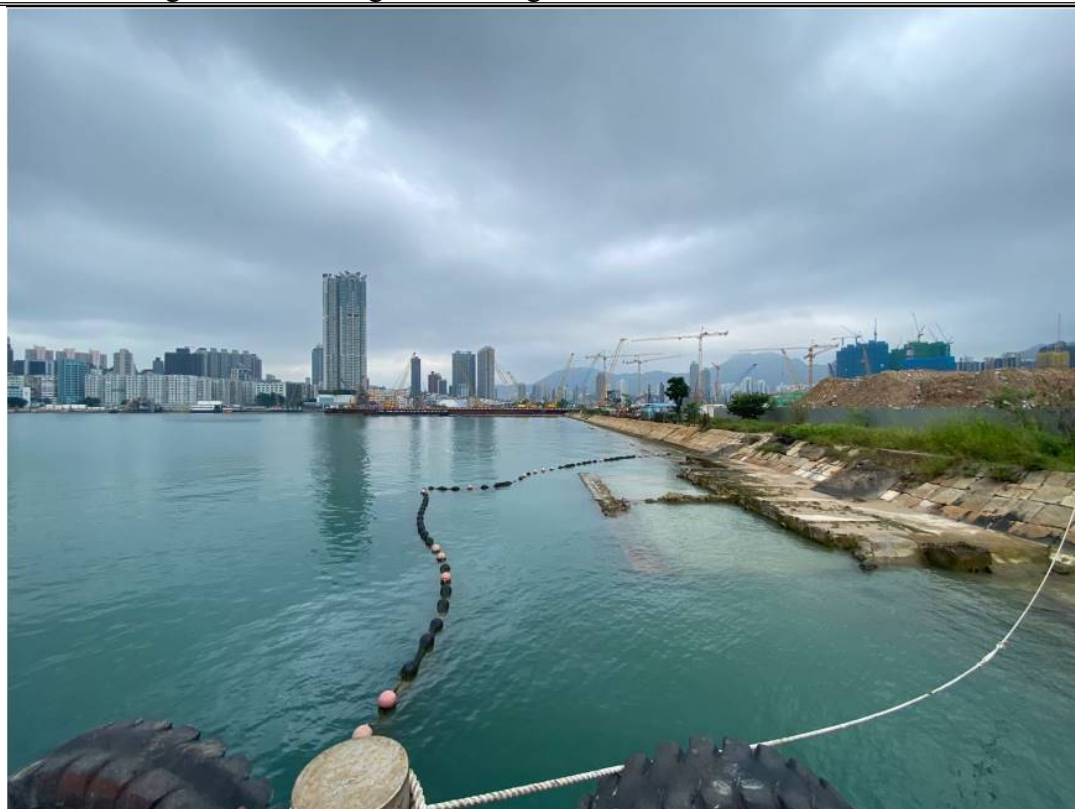
Photo 5: Deposition of Silt curtain near Barging Point.
