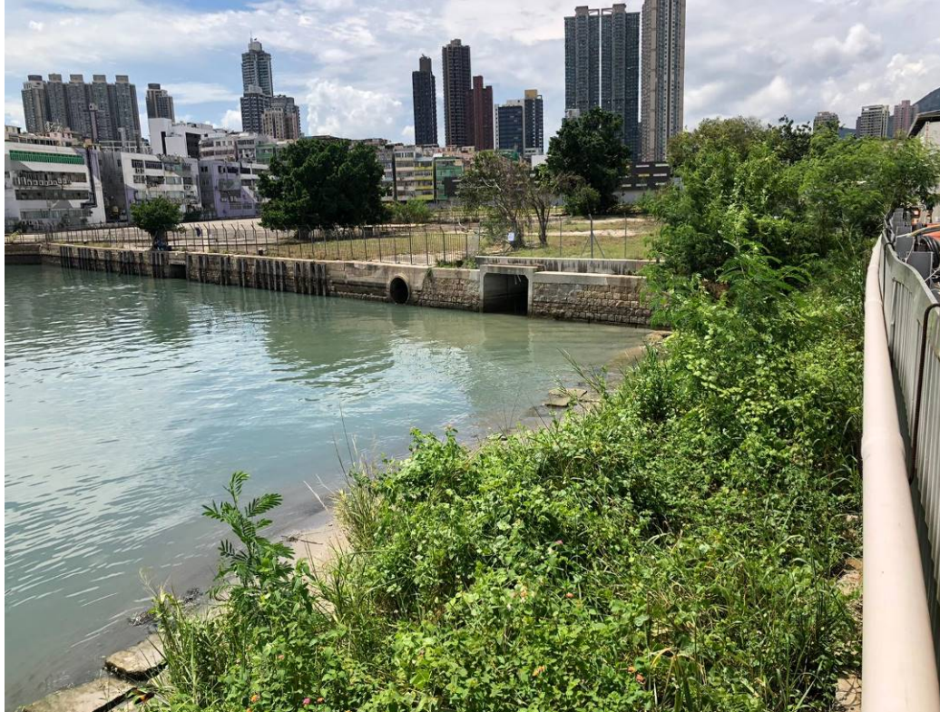
Photo 1a: Box Culvert near To Kwa Wan Typhoon Shelter (10 September 2020)
