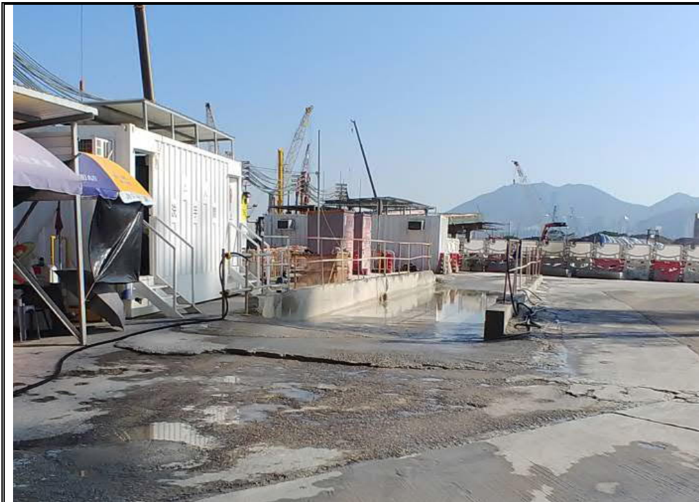
Photo 2: Wheel washing facilities at South Gate No. 3 (1 December 2020)
