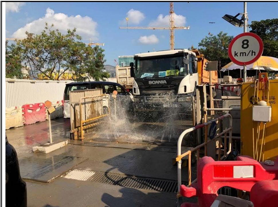
Photo 3: Wheel washing facilities had been provided and implemented at gate 3C
