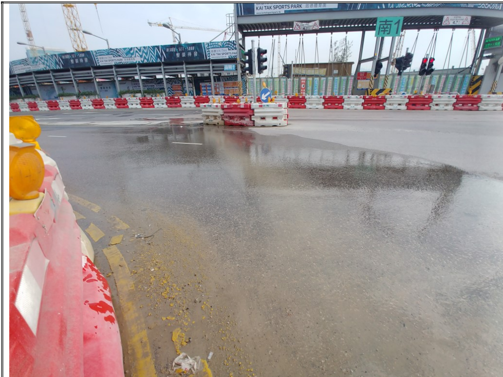
Photo 1c. Muddy water observed outside Gate N1 (8 December 2020)
