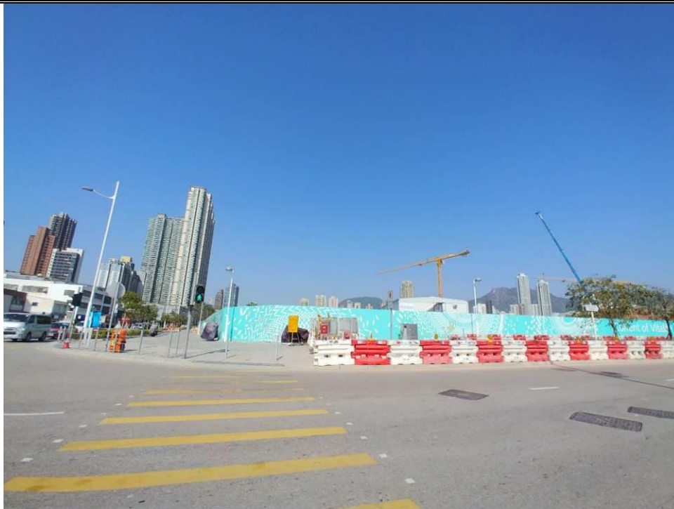
Photo 1a: Road condition at Shing Kai Road (Kowloon Bay direction) near Sung Wong Toi Road (3 February 2021)
