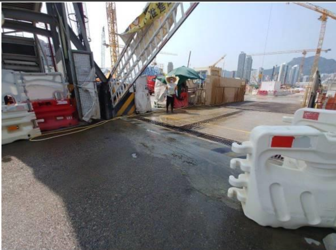
Photo 4: Cut off drainage was implemented at vehicle access. (26 March 2021)
