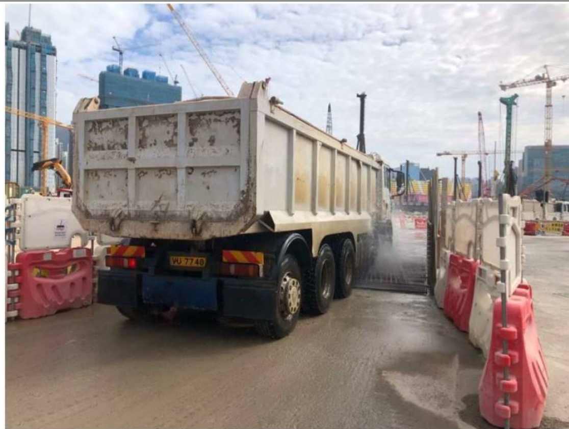
Photo 2: Wheel washing facilities have been installed and implemented at all site exits.
