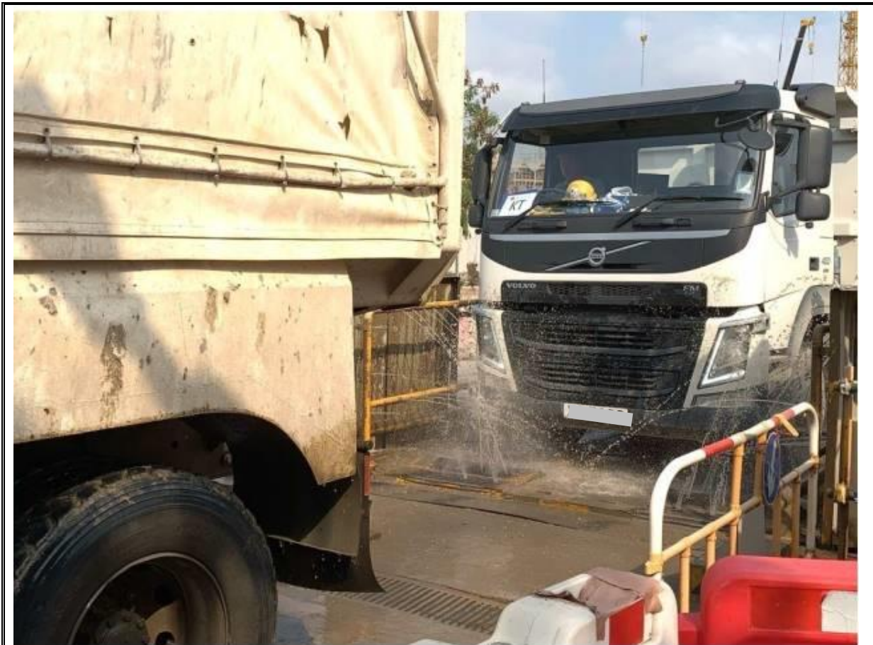
Photo 3: Wheel washing facilities have been installed and implemented at the vehicle access of haul road 3C. (15 March 2021)
