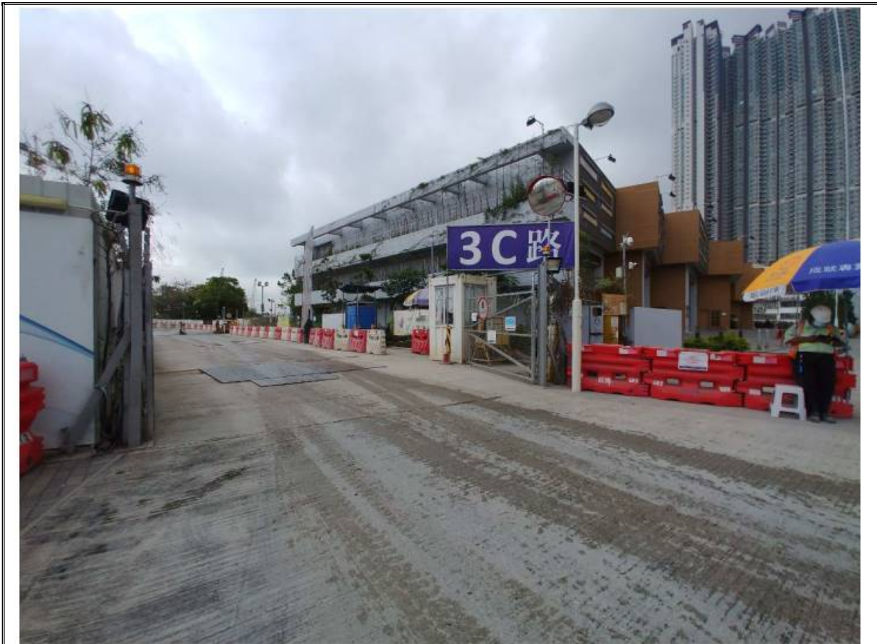
Photo 2: No slit contamination on nearby pavement road surface was observed. (14 April 2021)
