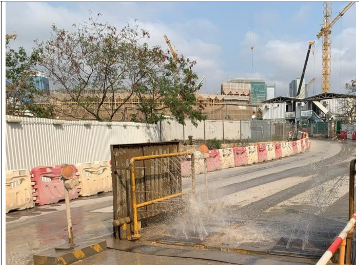
Photo 5. Wheel wash facility has been implemented at road 3C (19 April 2021)
