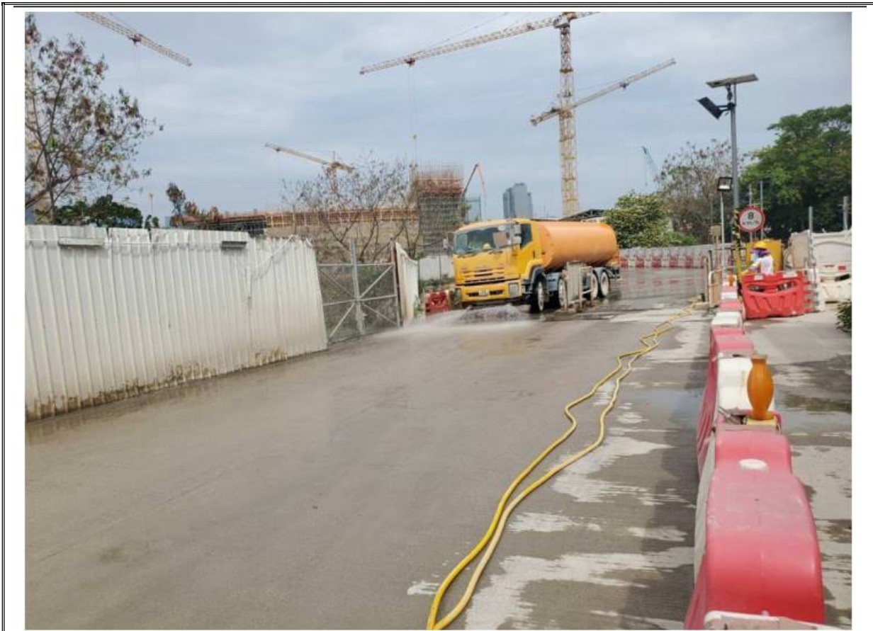
Photo 3: Water truck has been provided regularly at road 3C to remove all dusty material. (16 April 2021)
