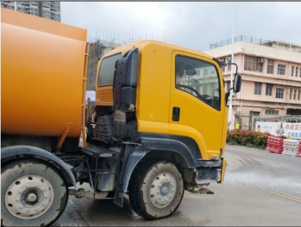
Photo 3: Water truck has been provided regularly at road 3C and entrance for dust suppression.
