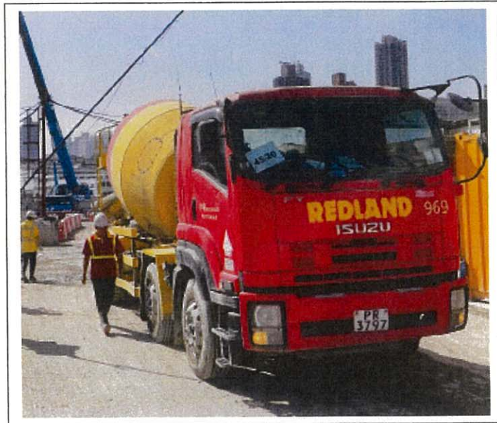
Concrete lorry mixer (Vehicle No. PR3797)
