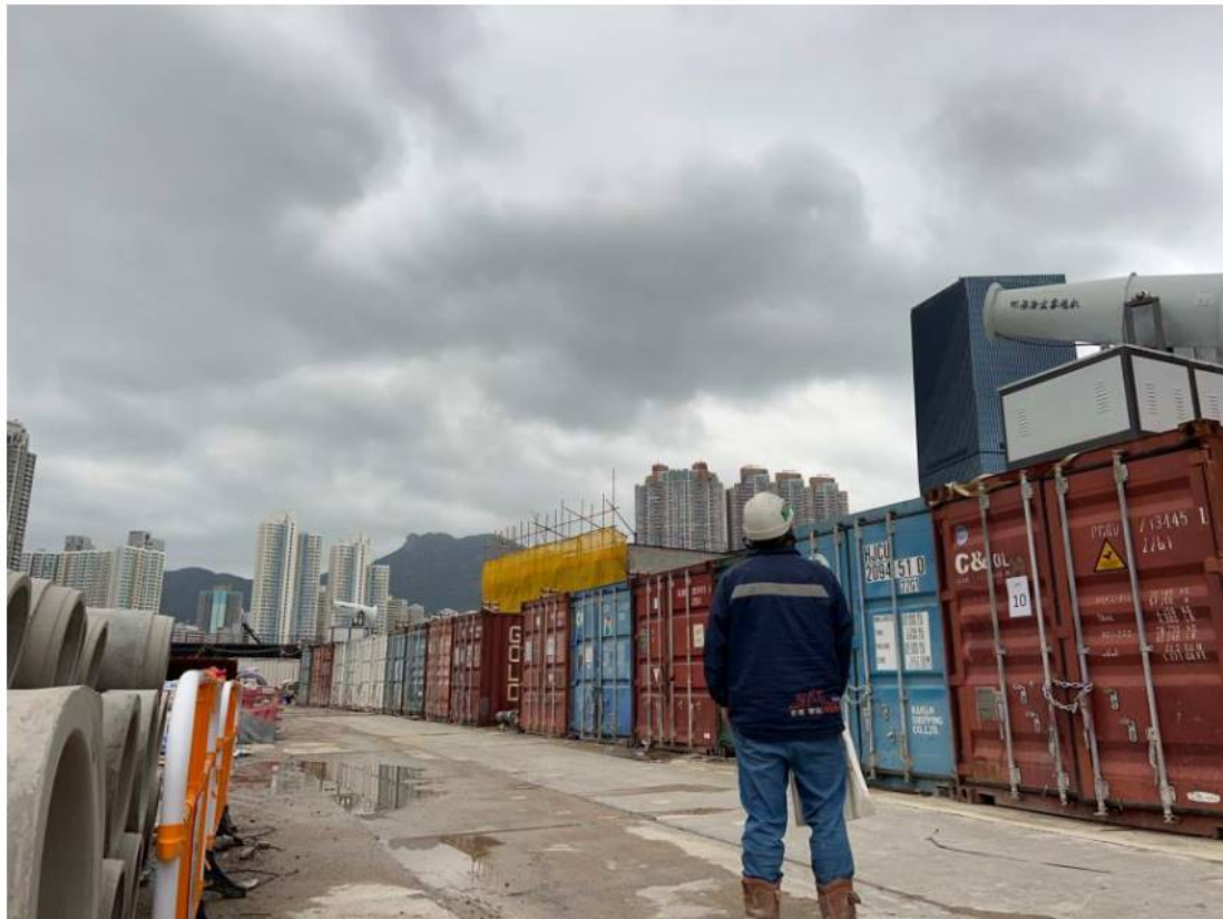
Photo 3: Site staff will be arranged for daily checking to ensure no operation of mist cannon by end of working day.
