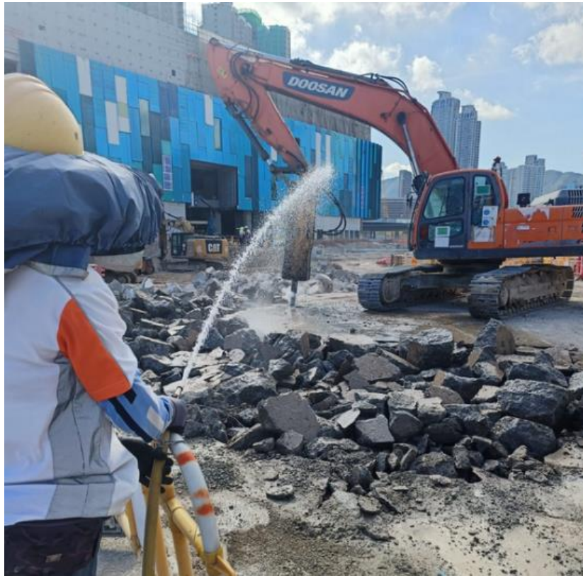
Photo 1: Water spraying had been implemented during ground breaking works.
