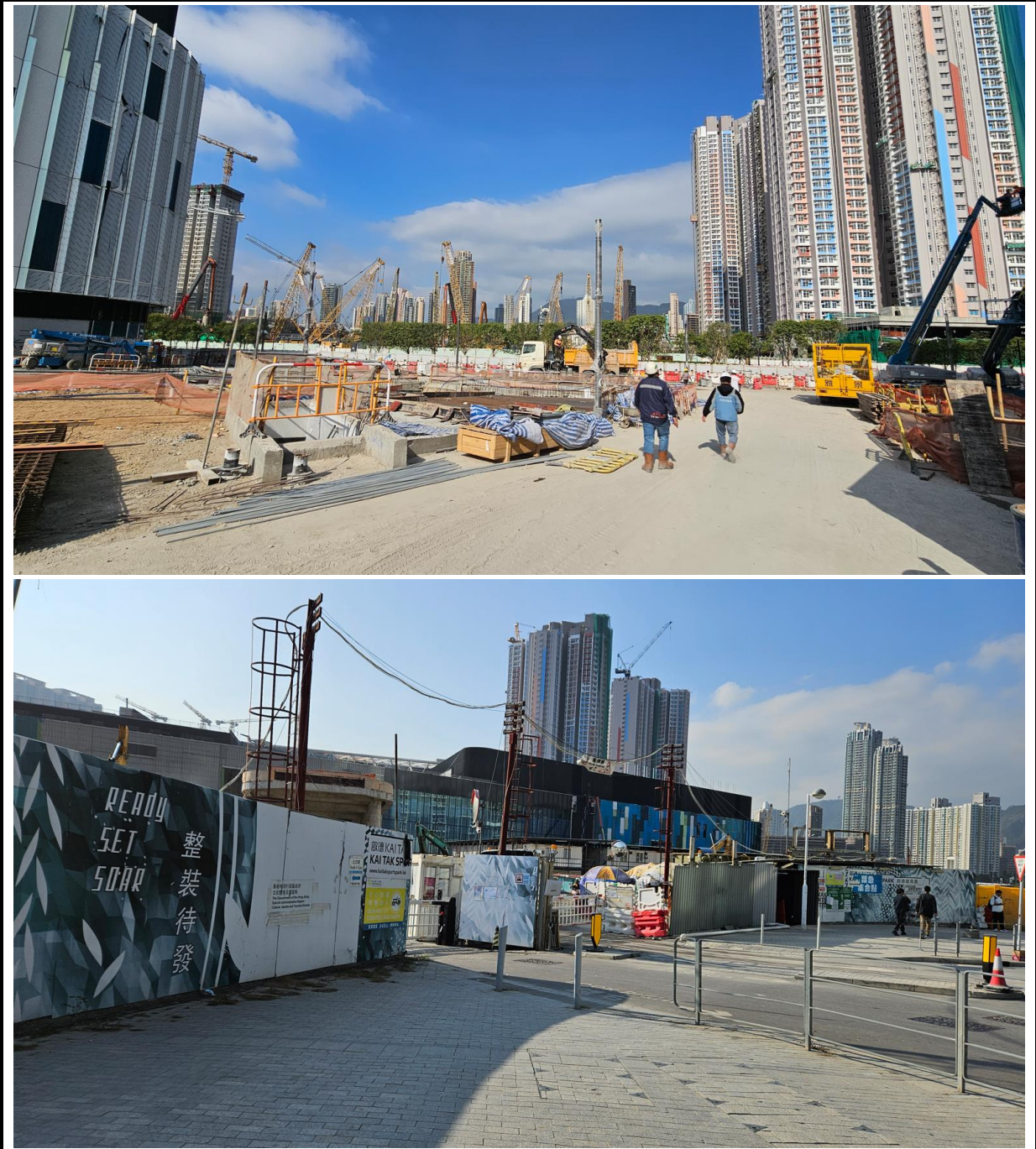
Photo 1a and 1b: Regular site inspection with contractor on 3 January 2024.
