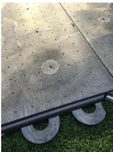
1. Proprietary turf protection system is placed over artificial turf
