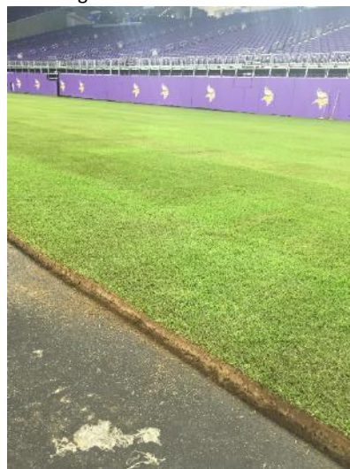
6. Completed section of 50 mm thick big roll turf
