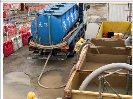
Photo 7a: Regular Sludge Removal at Sedimentation Tank
