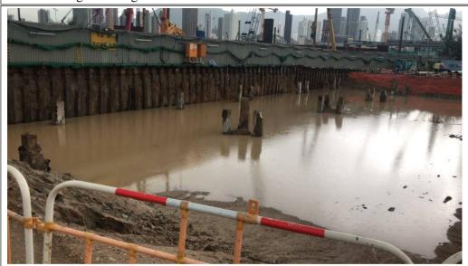
Photo 8a: Temporary Sedimentation Pond on Site
