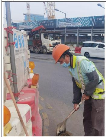
Photo 4: Worker to remove the residual sludge on road surface at Shing Kai Road(8 December 2020)
