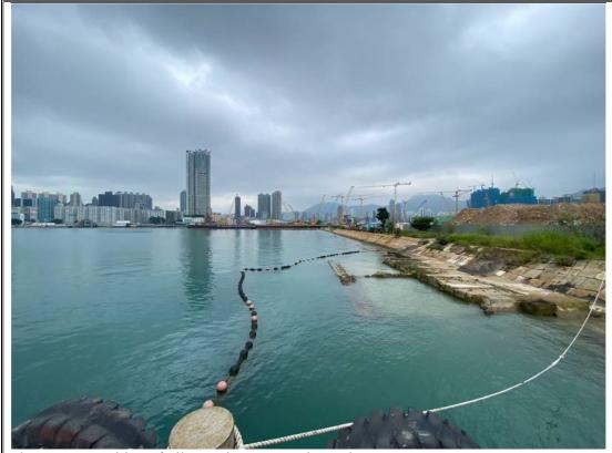
Photo 5: Deposition of Silt curtain near Barging Point.
