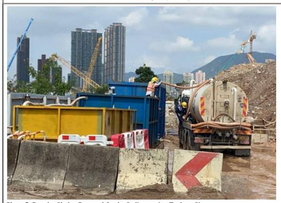
Photo 7: Regular Sludge Removal for the Sedimentation Tank on Site.
