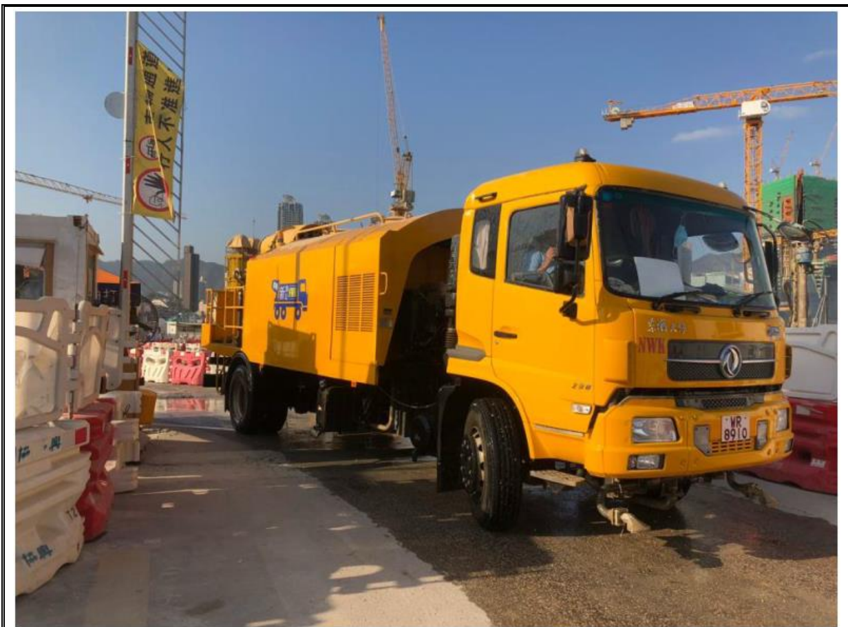
Photo 4: Water spraying by water truck has been suspended in front of North 1 Gate.
