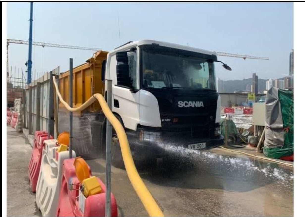
Photo 2: Wheel washing facilities were installed and implemented at vehicle access. (26 March 2021)
