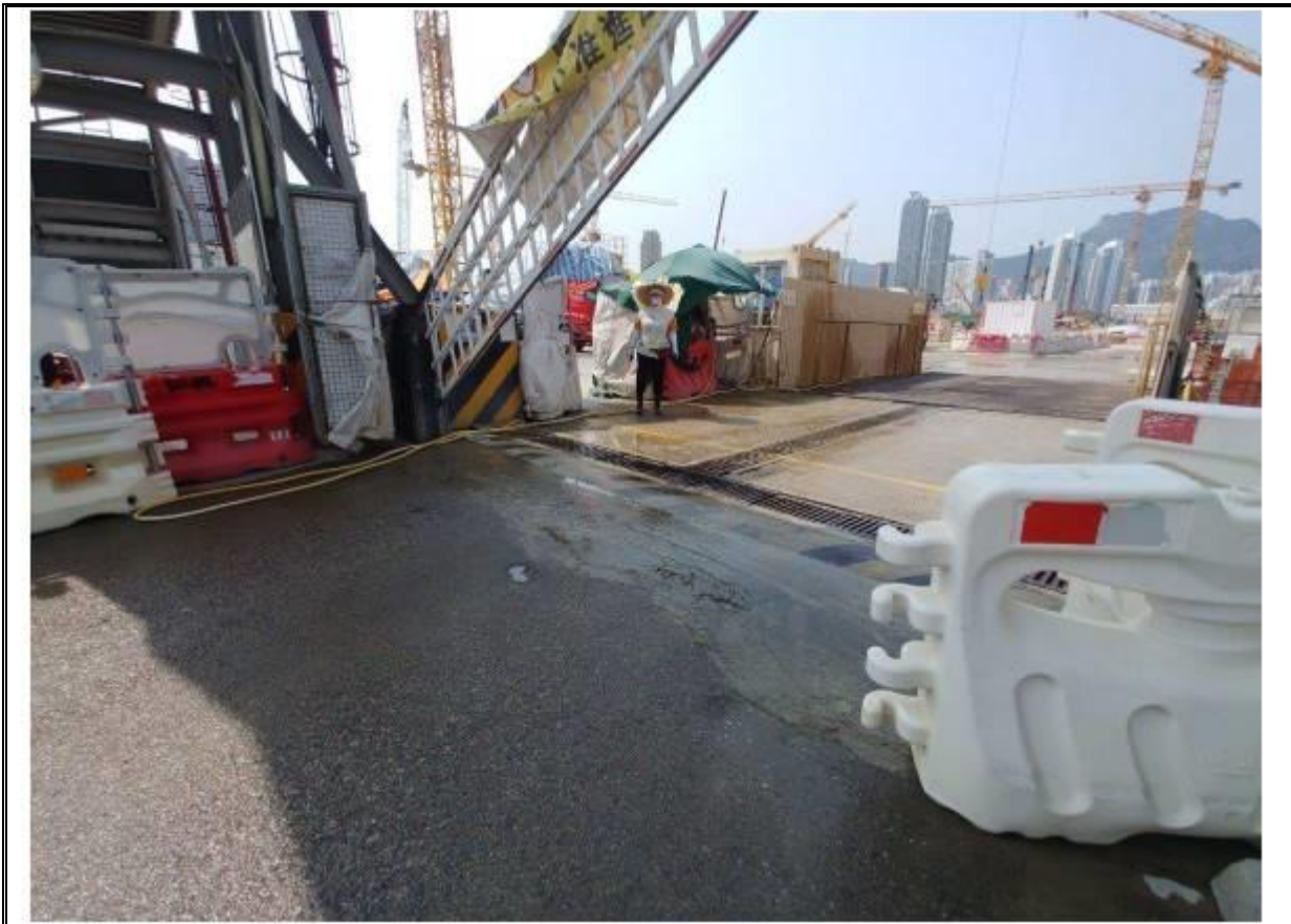
Photo 4: Cut off drainage was implemented at vehicle access. (26 March 2021)
