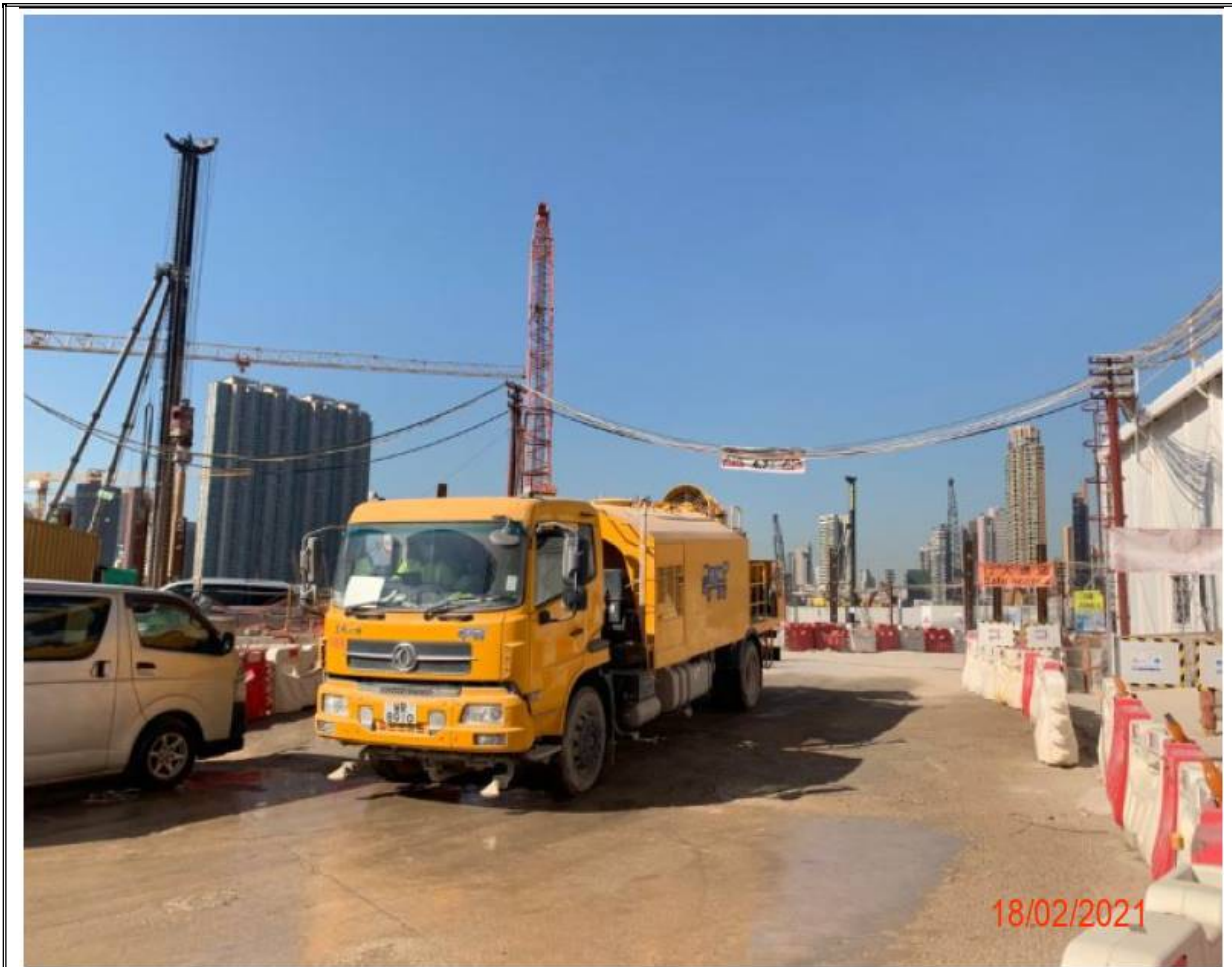
Photo 3: Regular water spraying by water truck has been provided to main haul road to ensure wet surface on site. (18 February 2021)
