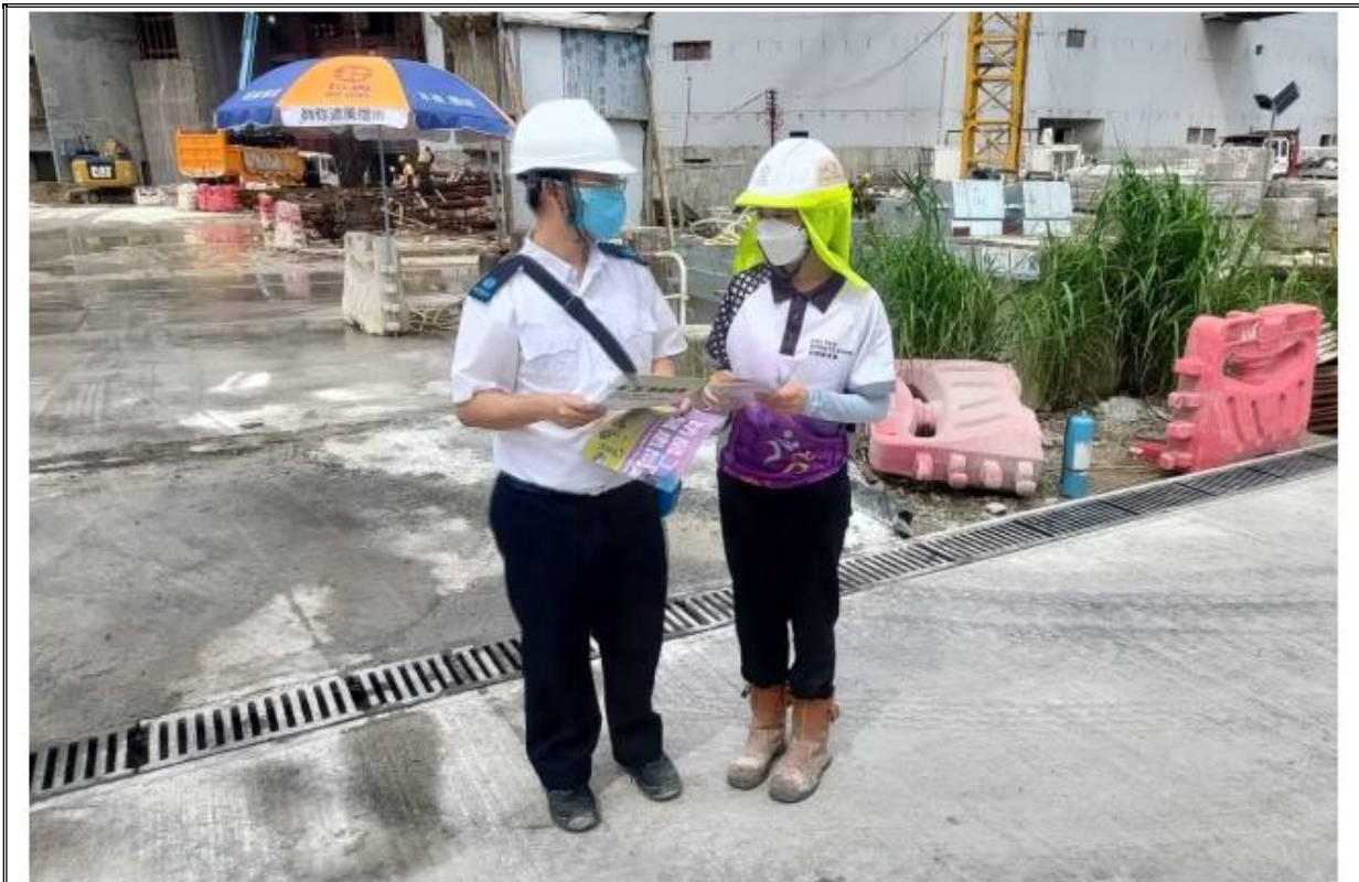
Photo 7: FEHD site inspection on 21 June 2022
