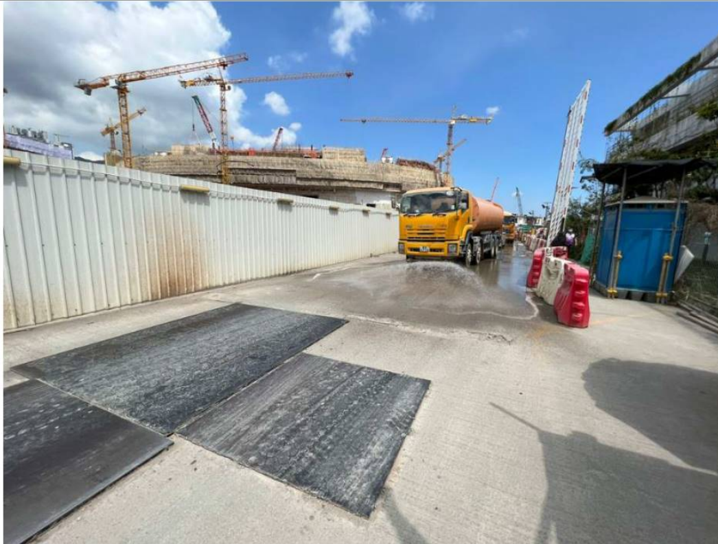
Photo 3: Water truck has been provided regularly at road 3C for dust suppression. (14 April 2022)
