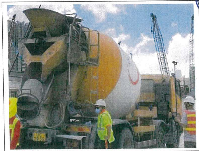
Concrete lorry mixer (Vehicle No. UC2932) 混凝土攪拌車 (車牌號碼 UC2932)
