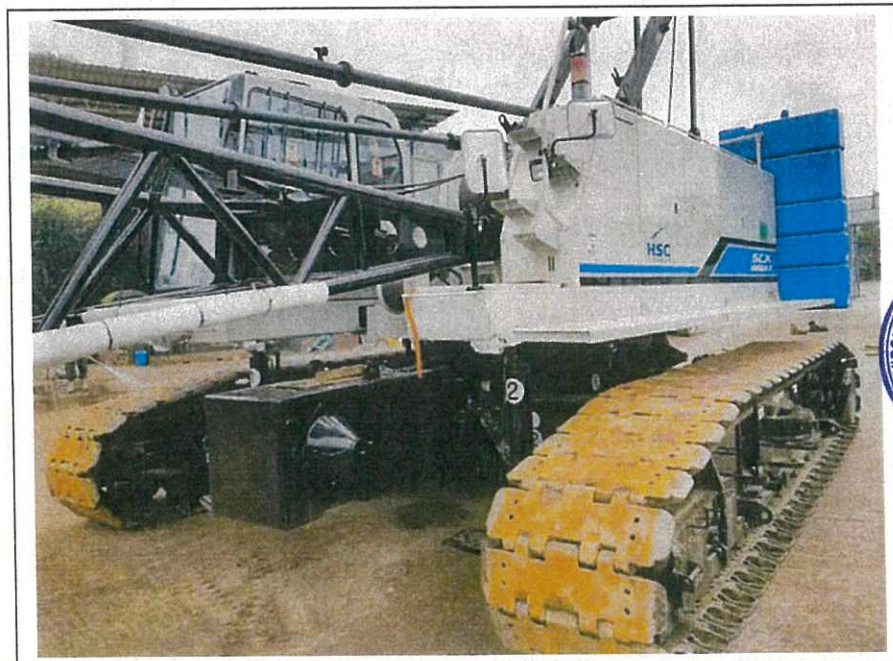
Crane, mobile (diesel), with Quality Powered Mechanical Equipment Label showing a Sound Power Level \leq 103 dB(A)
