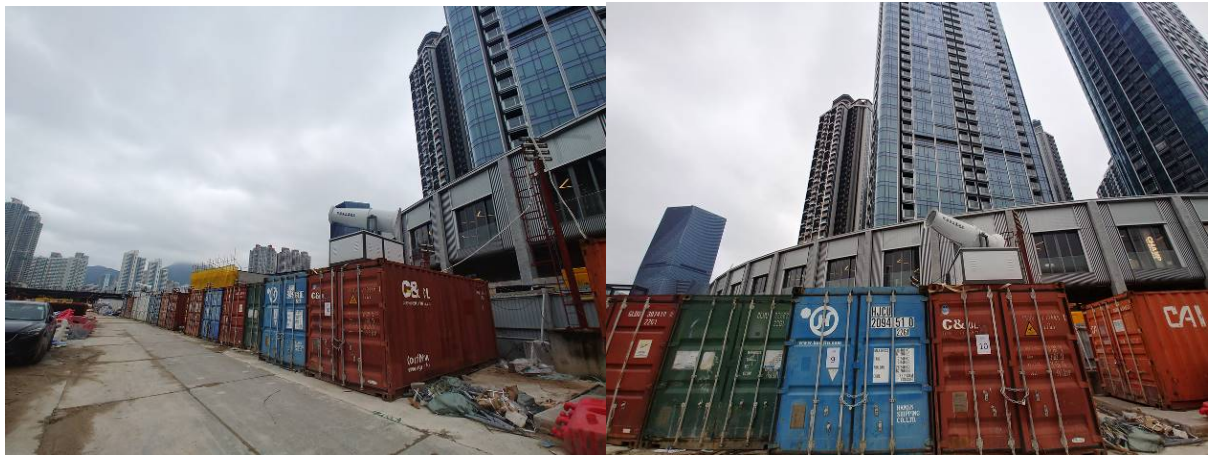
Photo 1a and 1b: Photo of mist cannon during site inspection on site on 28 March 2023. (site area close to the Muk Tai Street )
