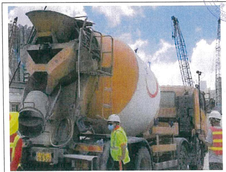
Concrete lorry mixer (Vehicle No. UC2932)
