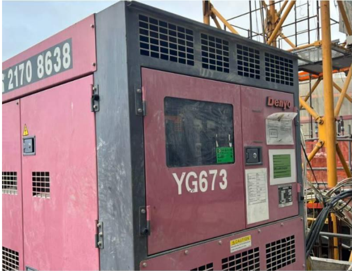
Photo 2: Power Mechanical Equipment with Quality Power Mechanical Equipment (QPME) labels were used at site to lower the noise nuisance to the nearby residents
