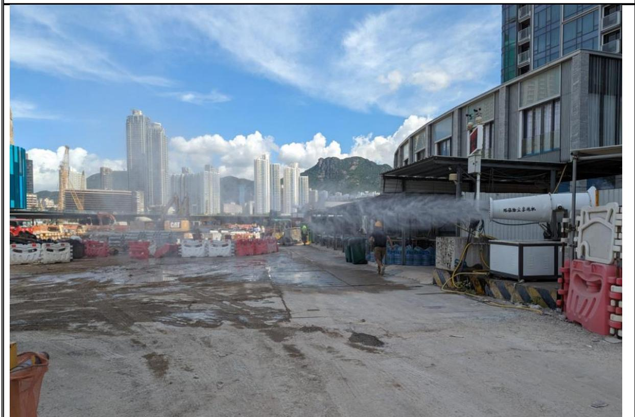
**Photo 3:** Water misting cannon had been installed to wet the area which water trucks cannot reach.
