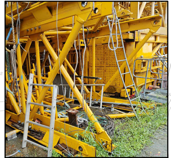
4_Storage of crane parts
