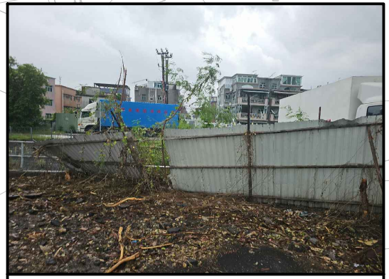
2_Southern part of E477 after Site clearance
