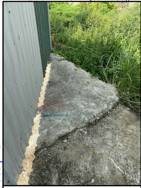
1_General view of site of E138 (view from the East)
