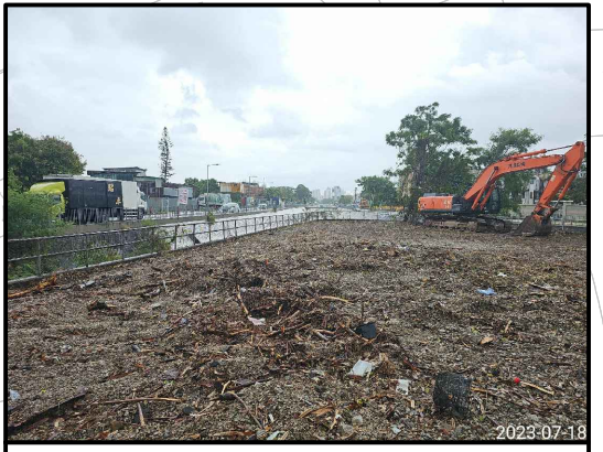
3_Northern part of E477 after Site clearance
