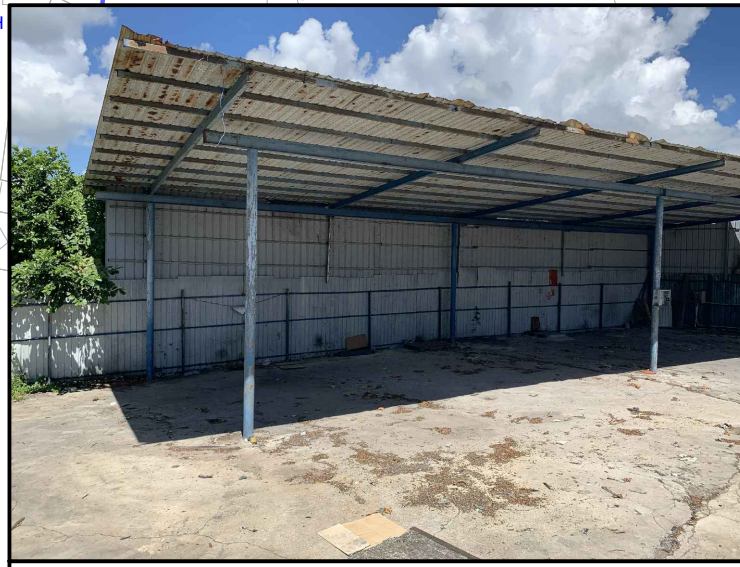
2_Eastern part of site with fully paved ground
