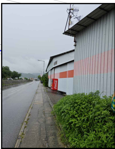
7_Temporary structure for warehousing at E119
