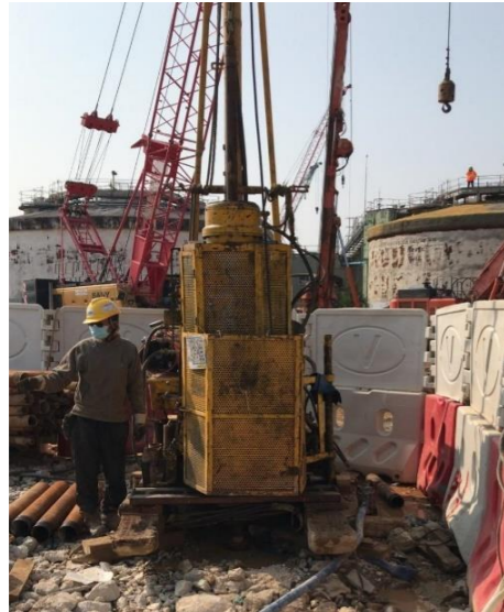
Preparation for Drilling
