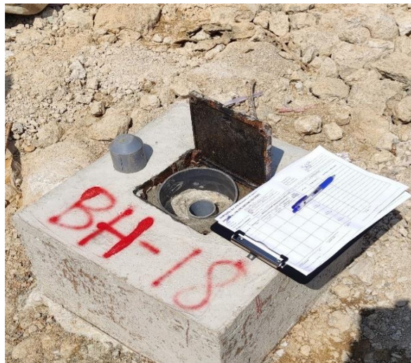
Set-up of Monitoring Well
