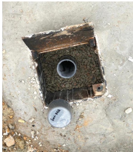
Set-up of Monitoring Well
