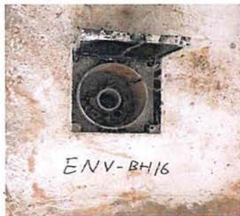
Set-up of Monitoring Well
