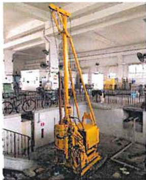
Preparation for Drilling
