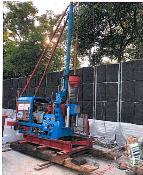
Preparation for Drilling
