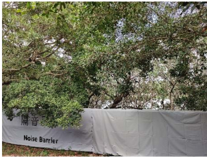
Acoustic mats placed along the fencing to San Pui River and rigid noise barriers in front of acoustic mats
