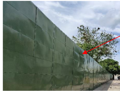
Acoustic mats placed along the fencing to San Pui River and rigid noise barriers in front of acoustic mats
