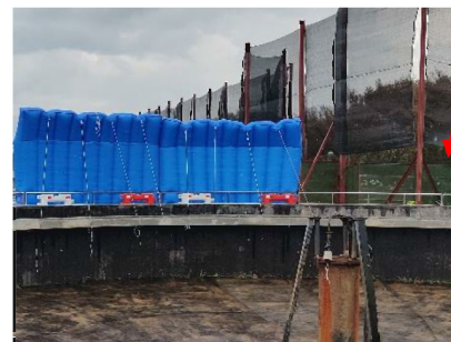
Acoustic mats placed along the fencing to San Pui River and rigid noise barriers in front of acoustic mats
