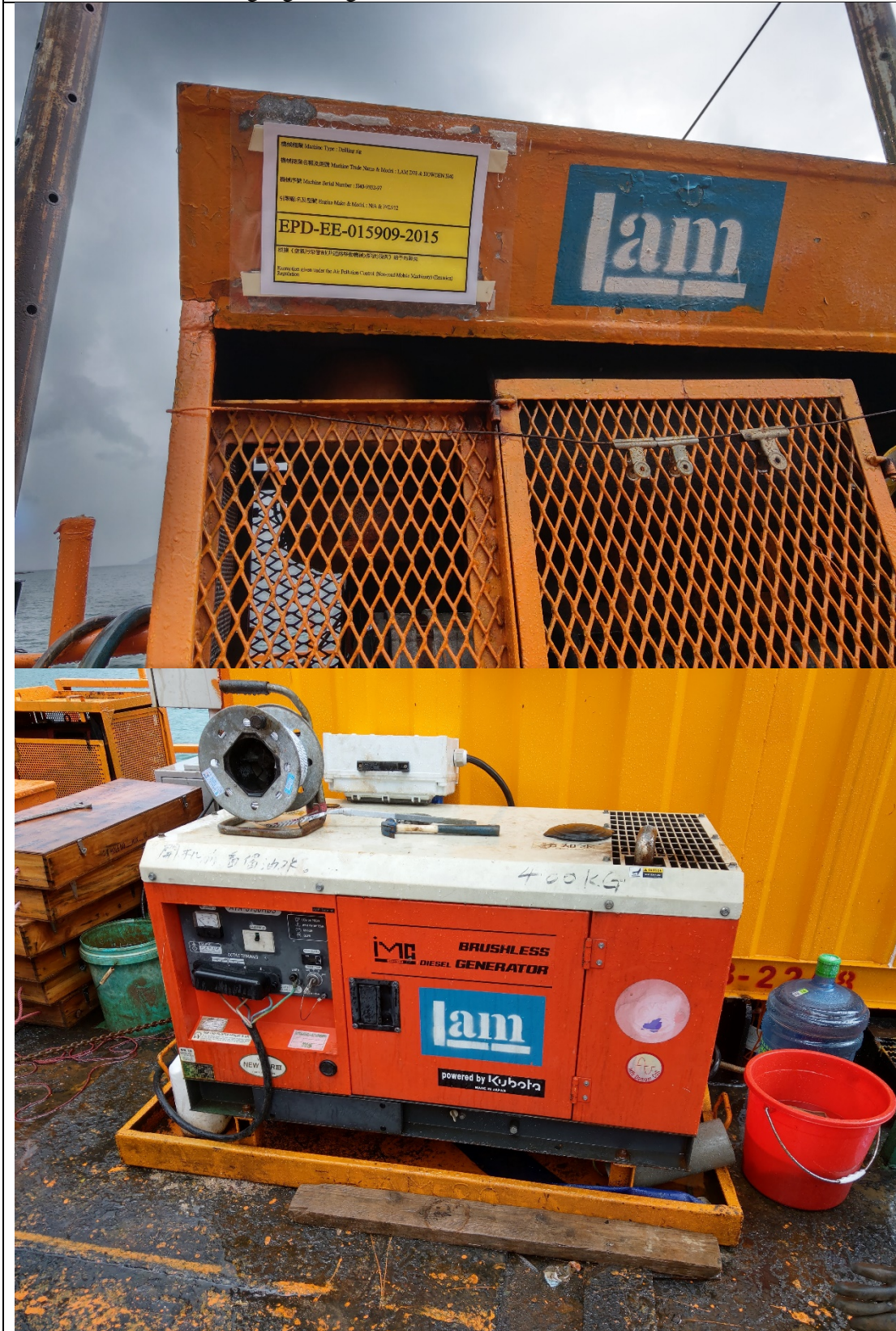
Good condition drilling rig and generator
