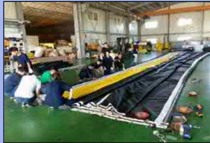
Fabrication of silt curtain
