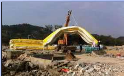
Handling of the silt curtain
