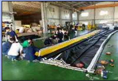
Fabrication of silt curtain
